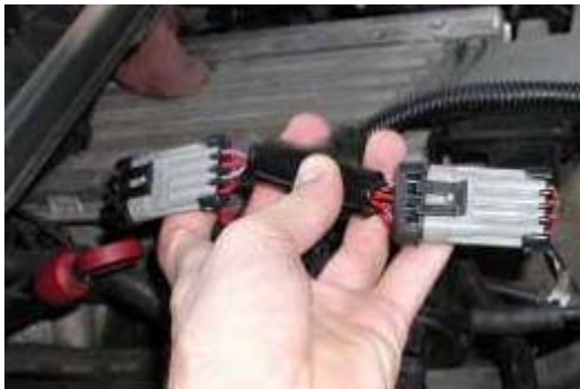
Figure 2: T-Harness Installed (1993-1996 Shown)
